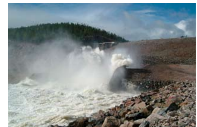
Changes in precipitation and water draining will impact on barrage safety for Swedish nuclear power plant barrages. WSP has worked on many assignments over the last 10 years dealing with barrage safety assessment and measures for increasing barrage safety. Here the Letsi nuclear power plant is being released as a test in the Lule river.
