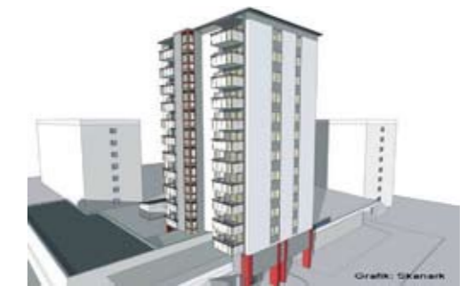
The first Swedish low-impact multi-family residential building, without a traditional heating system, was built in Karlstad in 2007. The building was constructed to be extremely energy-efficient and at the same time provide optimal indoor environmental quality. WSP projected and designed the climate shell as well as conducted the main construction of the building, on assignment by the municipal housing company KBAB (Karlstads Bostads AB). The architects were Skanark Arkitektbyrå in Karlstad.
