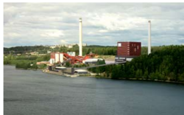
In 2009-2010, the new district heating plant at Igelstaverket will be the largest cogeneration plant (combined power and heating plant) run by renewable fuels in Sweden. It is owned by the energy company Söderenergi AB (part of the municipalities of Södertälje, Botkyrka and Huddinge). The new plant will reduce greenhouse gas emissions by 75 000 metric tonnes per year, which is equivalent of a reduction in greenhouse gas emissions from 25 000 new cars driving 15 000 km per year (the average distance for a Swedish passenger car). WSP is in charge of the construction management and is also contributing with expertise in fire & risk, land, and water & sewage management as well as with expertise in electrical systems. The photo montage was created by Scheiwiller Svensson Arkitektkontor AB.
