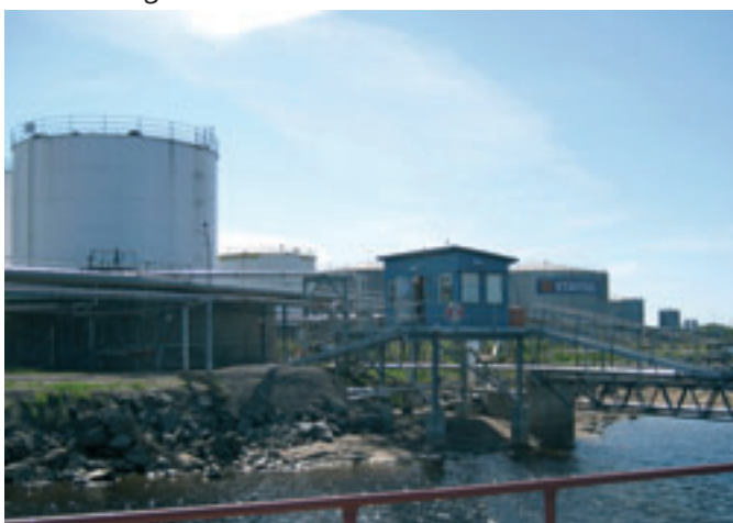
Work shed at the oil pier in Umeå Harbor
