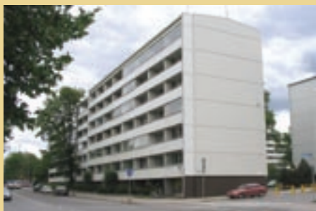
Martinsilta, Åbo, Finland Eurobor®treatment 2004 Client: As Oy Martinsilta
