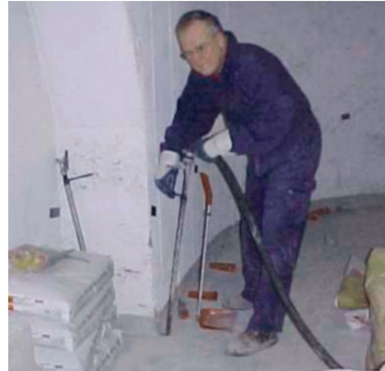
An injection sleeve is mounted in the borehole and EUROBOR® is pumped at low pressure.
