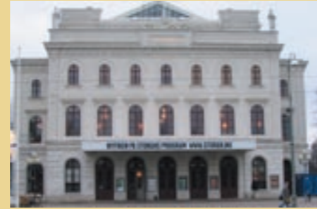
Stora Teatern, Göteborg Foundation inspections 86-91 Jerbor®treatment 1991 Client: KIGAB
