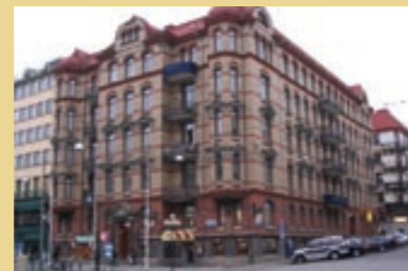
Kungssportsavenyn 27, Göteborg Foundation inspection 2004 Eurobor®treatment 2005 Client: Brf Lorensberg 57:1
