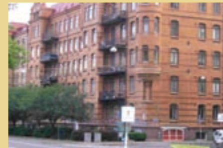
Södra Vägen 24, Göteborg Eurobor®treatment 2004 Client: ISS ECURO
