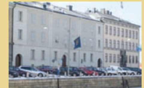
Länsresidenset, Göteborg Foundation inspection 2000 Jerbor®treatment 2000 Client: National Property Board Sweden
