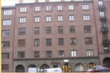
Eklandagatan 14, Göteborg Foundation inspection year 2005 Eurobor®treatment year 2006 Client: Brf Eklandagatan 14
