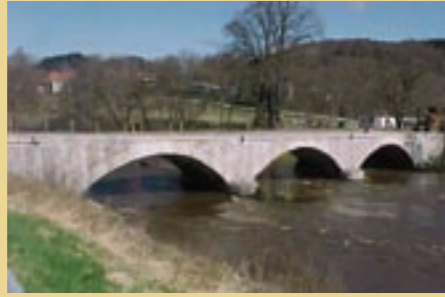
Kvistrumsbron, Munkedal Foundation inspection 1992 Jerbor®treatment 1993 Client: Swedish Road Administration
