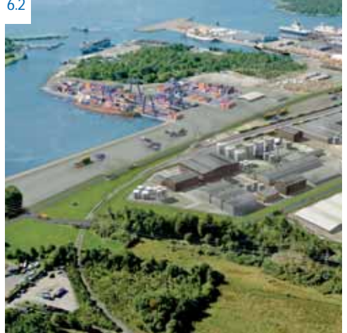
6.2 Port of Karlshamn Investigations and design for future development of the harbour including industrial estate and marshalling yard.
