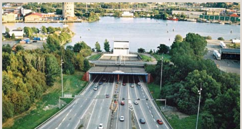
The Tingstad tunnel in Gothenburg.
